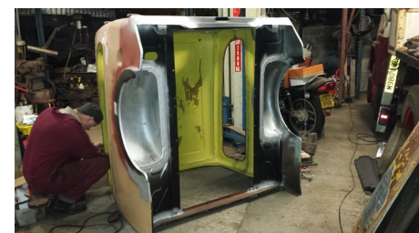
Cargo box being welded
